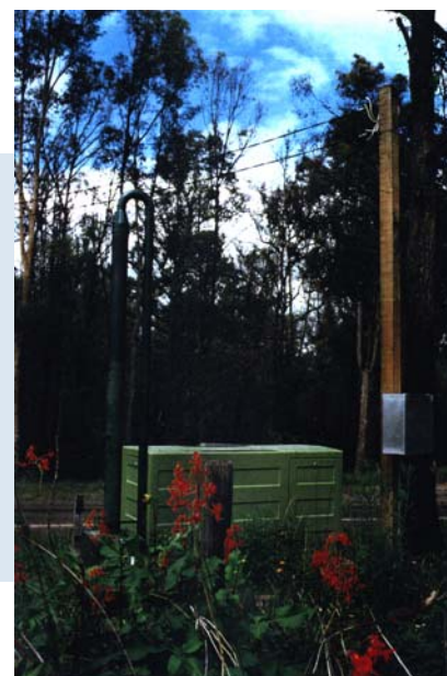
Sewer Vent Installation including optional enclosure.
